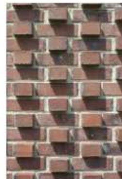
Example of brickwork proposed
