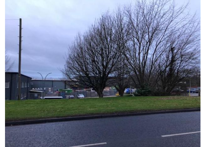
▲ Photo taking looking west from Merse Road towards rear of site showing the existing solar panels on building
