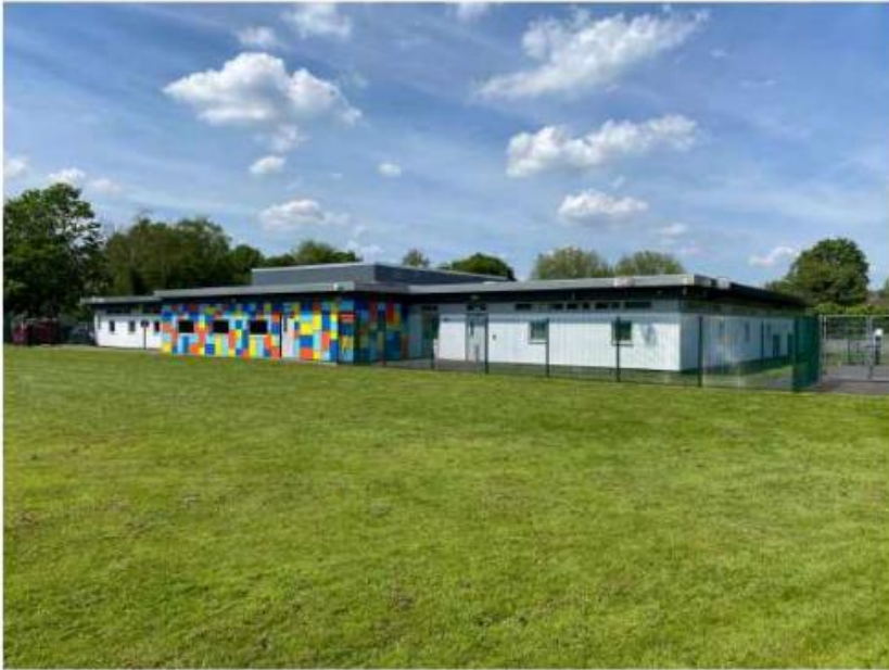
Existing Main School Building - Area 1
