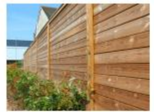
2.5m high timber acoustic fencing
