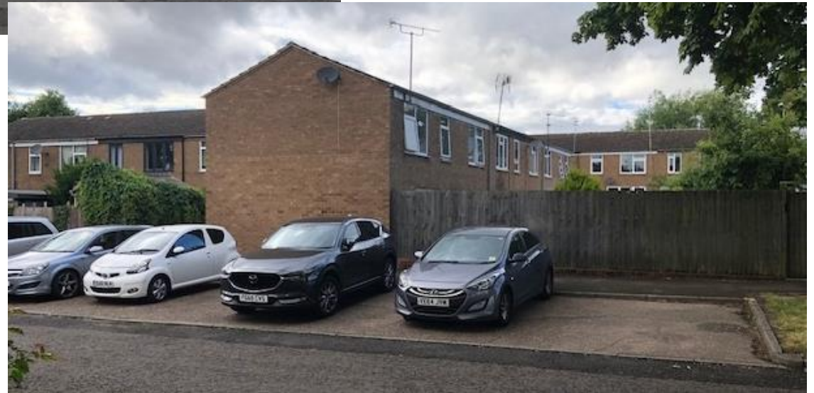
Row of parking to the south of the site
